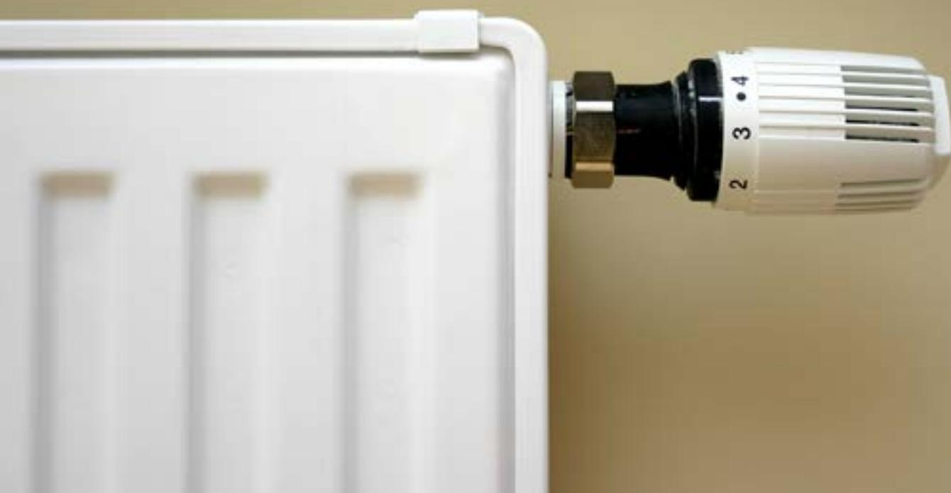
**Fitting Thermostatic Radiator Valves (TRVs) is the most efficient and effective way to control the temperature of the home. They work in conjunction with boilers timers and wall mounted room thermostats and are a simple and affordable way of controlling the heat output of a radiator and the temperature of a room.**
